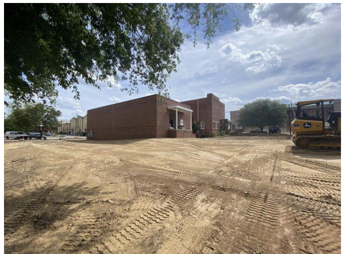
Preparing for paving
