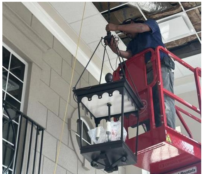
New decorative lanterns being hung in the lobby
