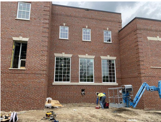
Three large windows installed in the visitors gallery
